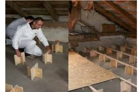
pose double plancher
